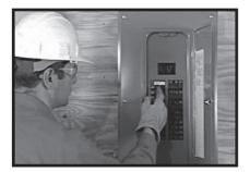
Check to be sure that voltage and frequency from the generator is correct. If line-to-line voltage is not 240 volts, refer to the Installation Guide for the proper adjustment procedures. If line-to-neutral voltage is not 120 volts, check the neutral connection between the generator and transfer switch.
